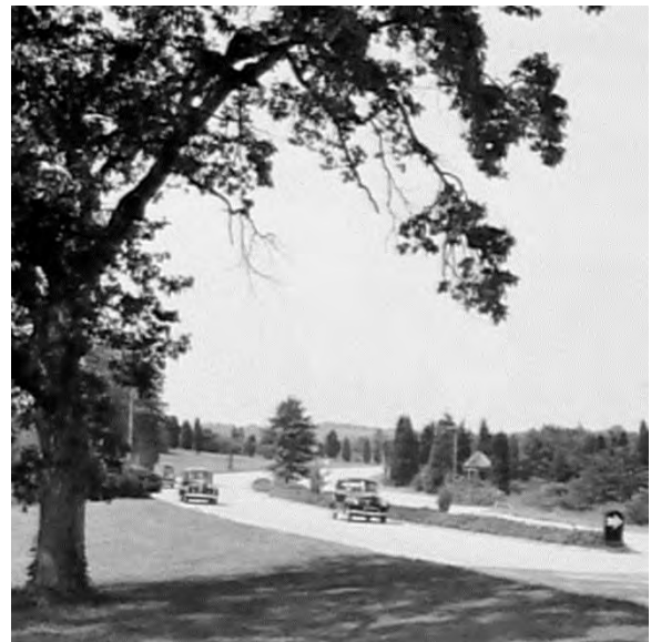
Figure 15. One Red Oak in Median (National Archives Photo No. 30N-45-1522)
