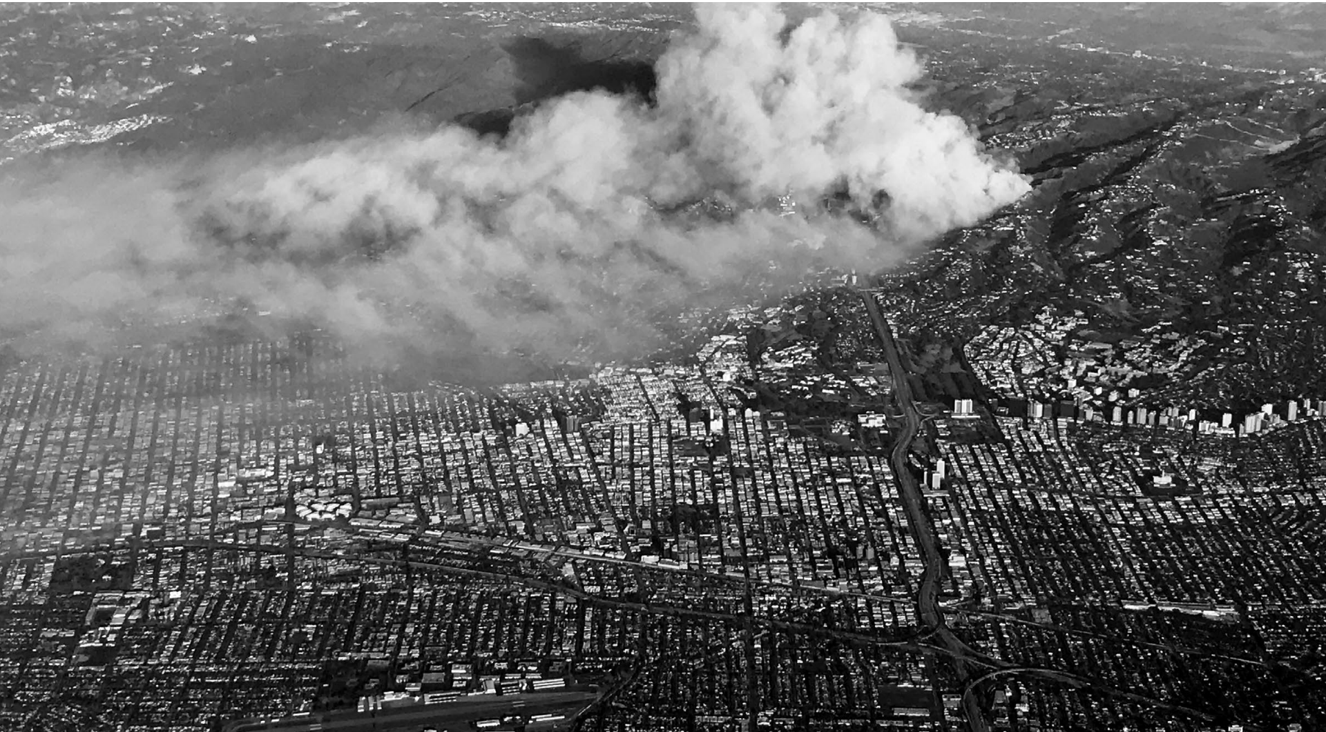
Aerial view of a wildfire in Los Angeles Photo: Bethany via Adobe Stock
