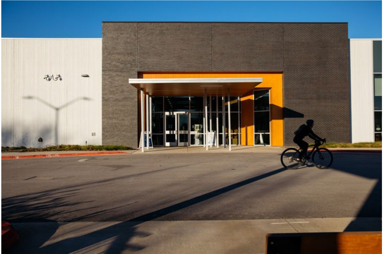
Barret rides her bike through the parking lot in front of one of the first buildings to be completed and operational on the new Walmart campus in Bentonville. Photographer: Terra Fondriest/Bloomberg
