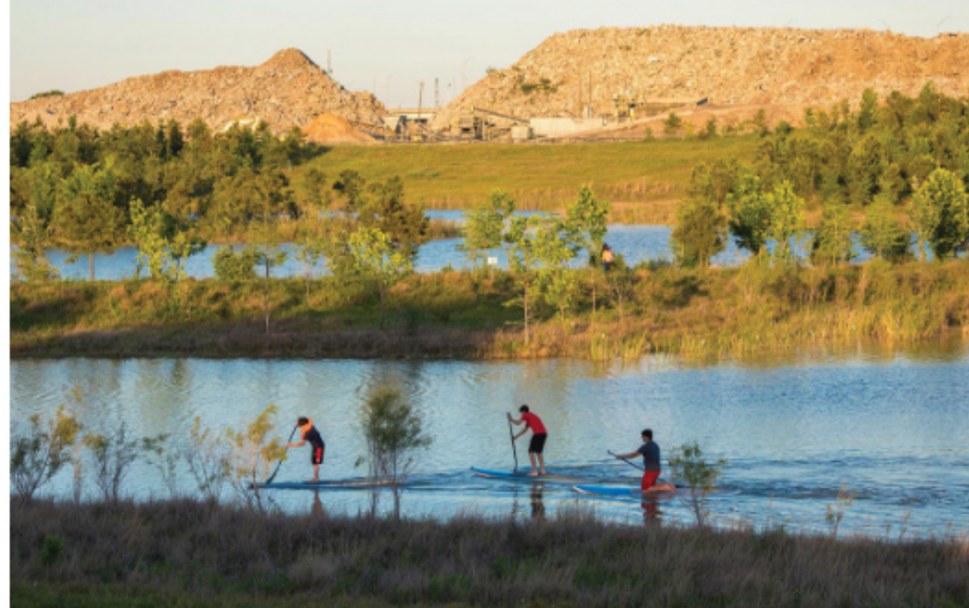
SWA Group helped the Harris County Flood Control District create a series of interconnected man-made lakes in southwest Houston. Known as Willow Waterhole, they reduce flooding by storing excess stormwater. Photo © Jonnu Singleton, click to enlarge.
