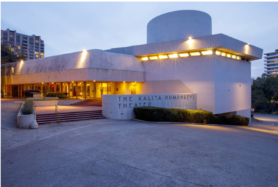
Frank Lloyd Wright's long-neglected Kalita Humphreys Theater is still moldering along Turtle Creek after a conservancy formed to save it was foolishly rebuffed by the city. (Smiley N. Pool / Staff Photographer)
