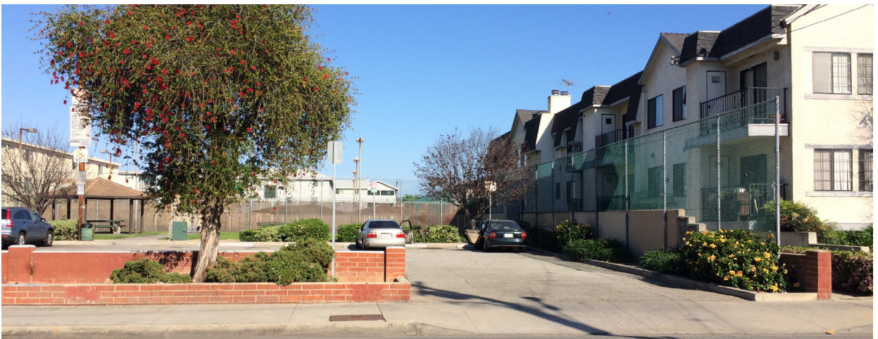
The existing park conditions, with parking lot, picnic table, and permanently locked tennis courts.
