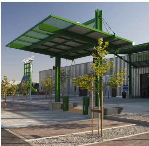
Main entrance showcasing sustainable site features
